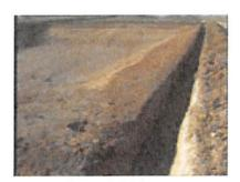
**Step 1**- Set the anchor trench approximately 3.00′ (0.91 m) back from the top of the slope.
