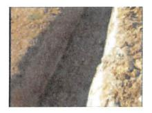
**Step 2**- Check to make sure the transition at the top of the anchor-trench wall, nearest the slope, is free from protrusions.
