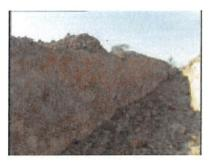
**Step 3**- Have an engineer use a pull out calculation to determine what size anchor trench is required. Without a pull out calculation, a typical anchor trench is 1.00′ (0.30 m) wide and 2.00′ (0.61 m) deep.
